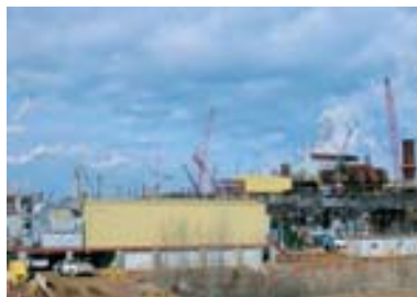
F35 72 kV integrated solution in pre-engineered building for Oil & Gas
