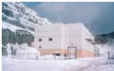
GIS in severe conditions.
