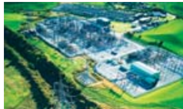
T155 400 kV GIS extension because of space requirements.
