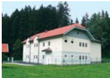
Full integration in surrounding to meet esthetic requirements with better public acceptance in a tourist area.
