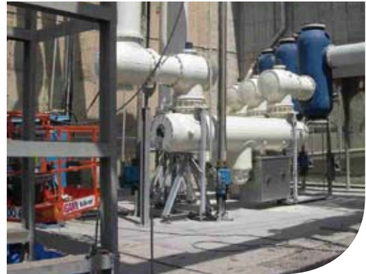
T155 circuit breaker: latest generation adapted to existing substation.
