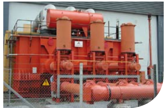
750 MVA 425 kV Power Transformer
