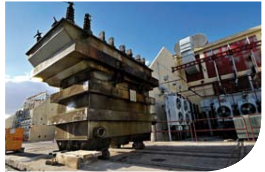
Turnkey power transformer removal/revamping
